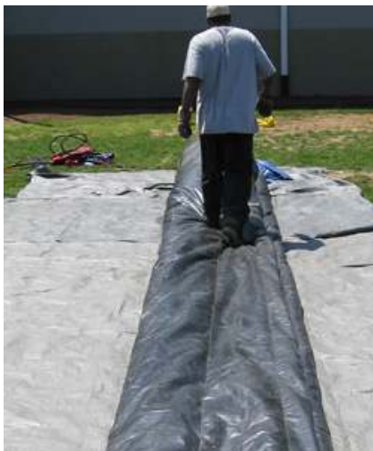
Step 2-6: Fold the Inflatable in 2-3 feet lengthwise and walk out air towards Ports (Blower tubes).
